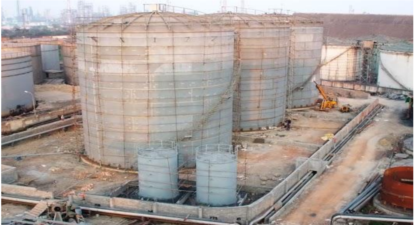
Haldia Liquid Storage Terminal Picture
