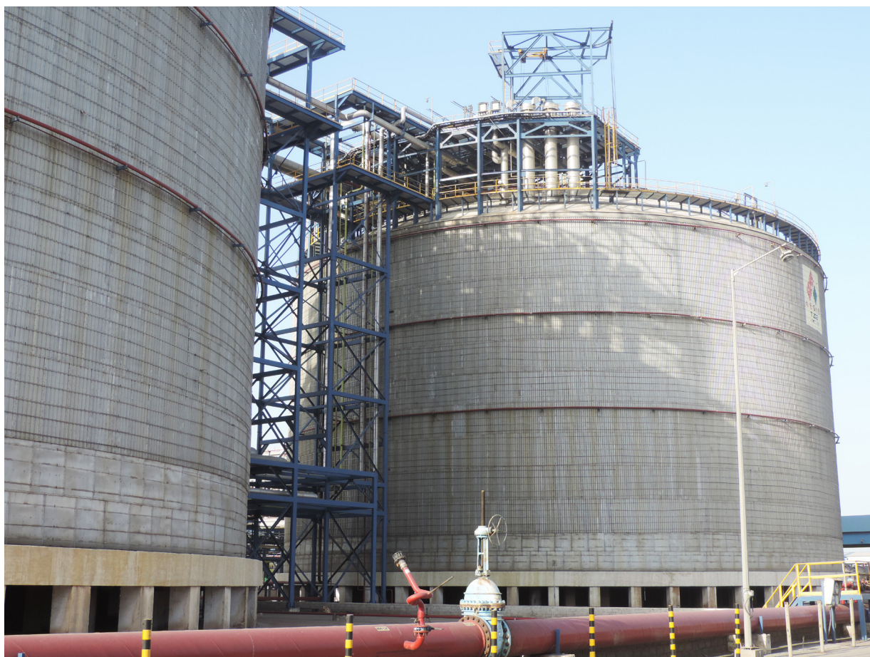
Close-up of LPG tanks at Kandla terminal
