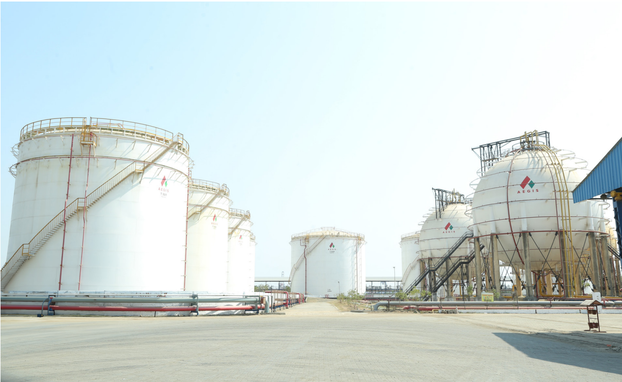
Liquid and LPG tanks at Pipavav terminal
