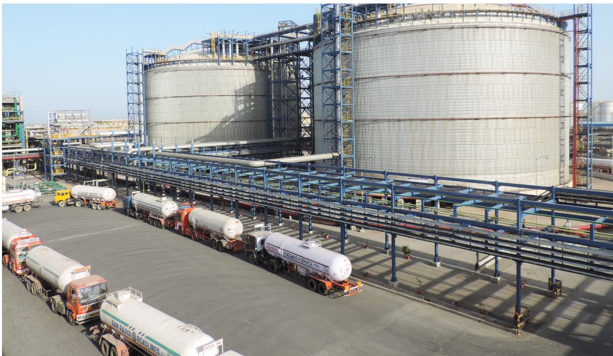
New Kandla LPG terminal
