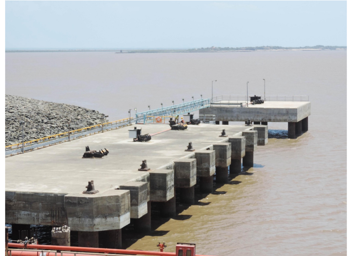
Pipavav Jetty infrastructure upgrade
