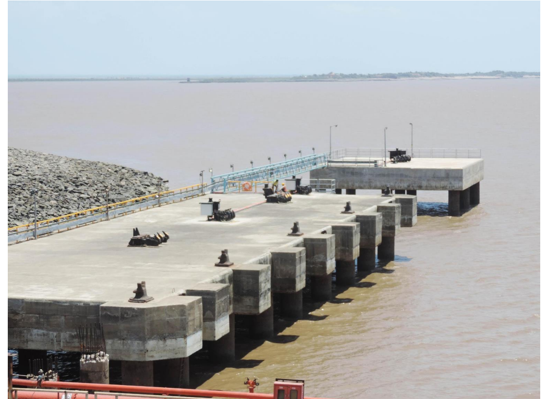
Pipavav Jetty infrastructure upgrade
